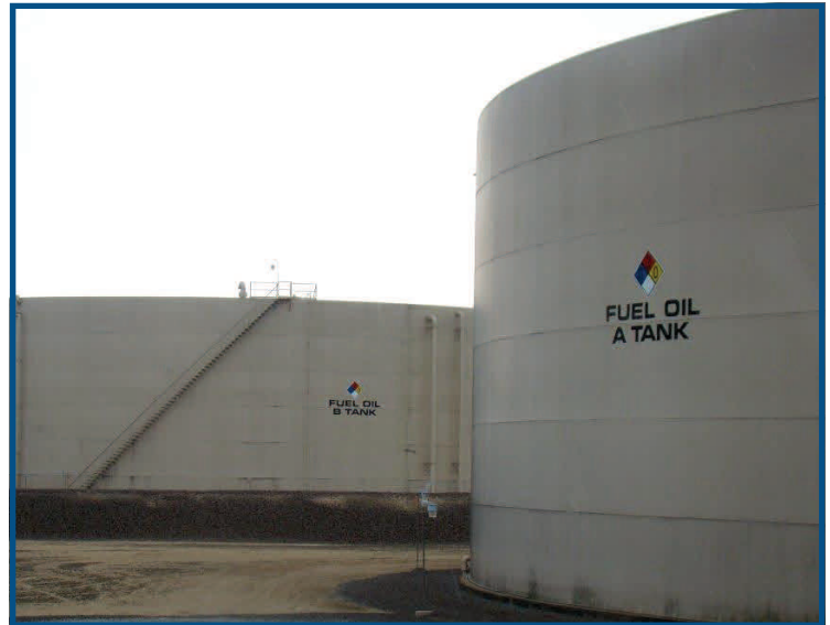
Stony Brook has 17.3 million gallons of oil storage capacity, primarily in the plant's two, 8.4-million gallon oil tanks, above.
